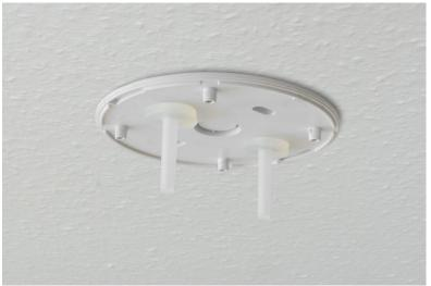
To fix the base plate, put the two silicone rings on the "sensor tubes" and push them all the way up. The base plate should now hang firmly on the ceiling.
