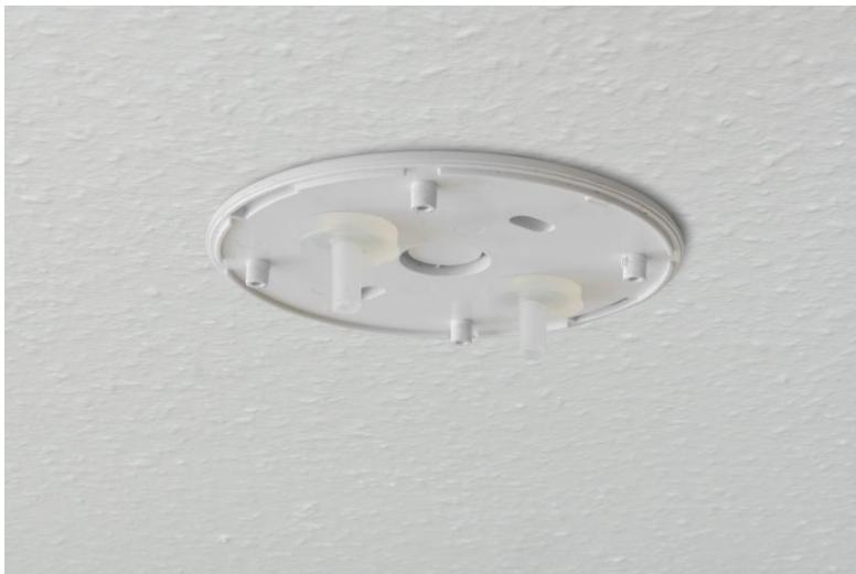
Cut off the two ends of the "sensor tubes" so that they are no longer than 10 mm from the base plate.
