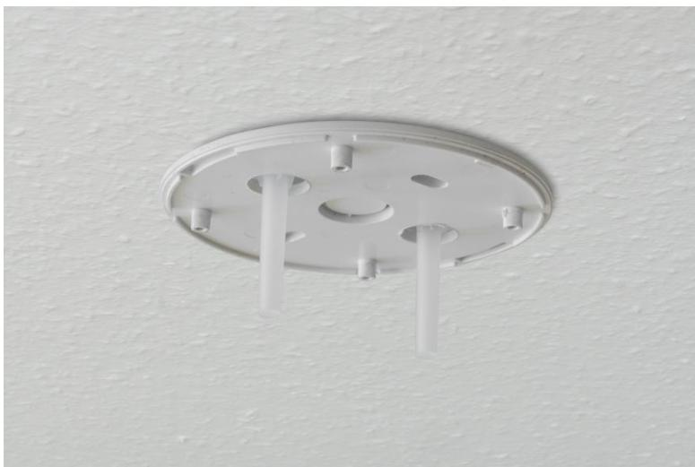
First guide the "sensor tubes" of the dew point sensor through the two large openings in the base plate. The smooth side of the base plate should face the ceiling.
